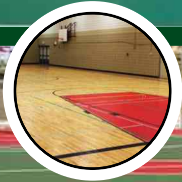
WOODEN INDOOR FLOORING
